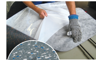
Acrylic Adhesive layer Protective layer
