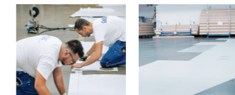
We weld carefully
